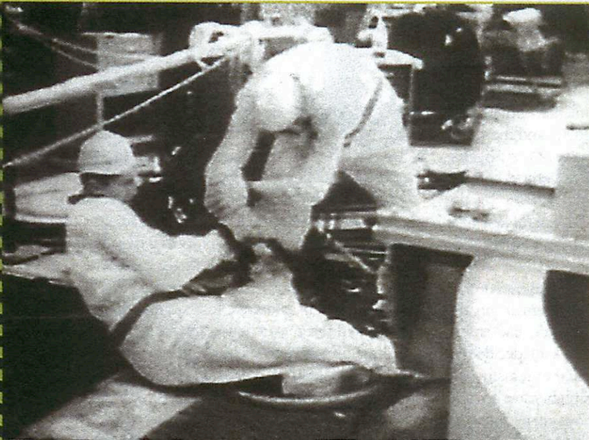
After the meltdown, Atomic International technicians John Pace (left) and a colleague adjust the reactor core lid so they can look inside to retrieve radioactive pieces of fuel elements. During the accident, levels of radiation were so high they could not be measured by instruments in the control room (below).
