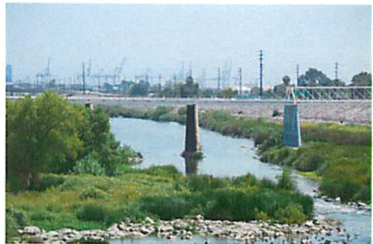
Willow Street, where odor and muck is very unpleasant, but greenery is finally in sight.
